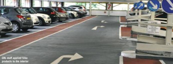
preferred option for the ramps, turning circles and the remainder of the car park decks. The Sika system was selected on account of its durability, cost effectiveness and fast curing properties that allow critical areas to be trafficked after four hours. This enabled circulation to be maintained in the car park, which remained operational throughout the works.
